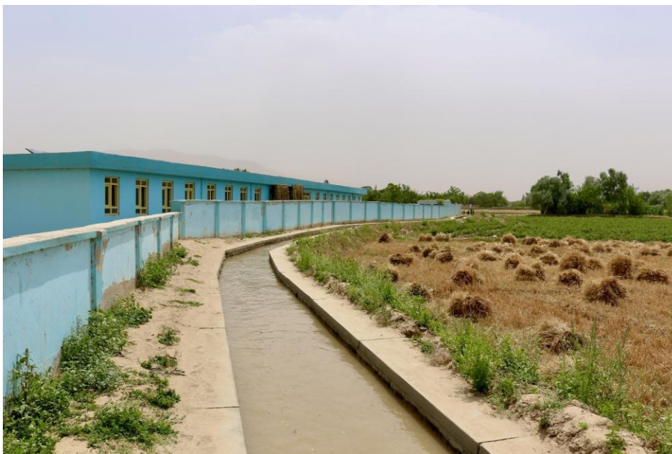
Canal lining infrastructure in Baghlan, northeastern Afghanistan. In addition to supplying water, it safeguards a local school from the destructive flooding that occurred every year. @UNDP Afghanistan/Edris Alamyar
